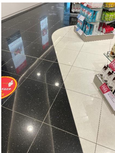
Figure 7: Flooring in shopping area
