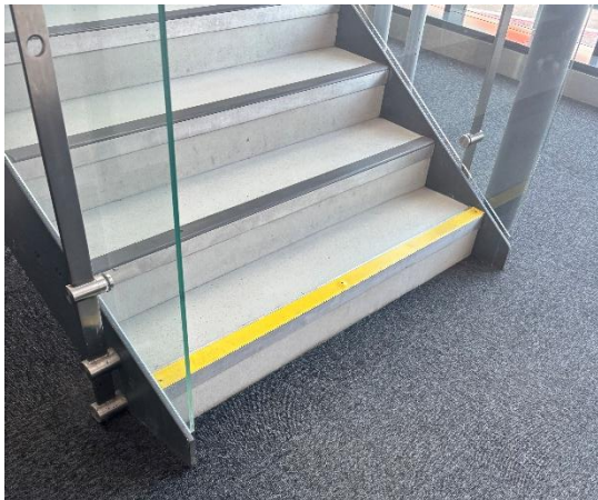
Figure 2: Yellow Strip on Staircase
